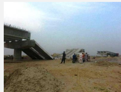
Overturning of newly launched girders of bridge on Ghan Stream, Jhelum, 22 nd May, 2016
