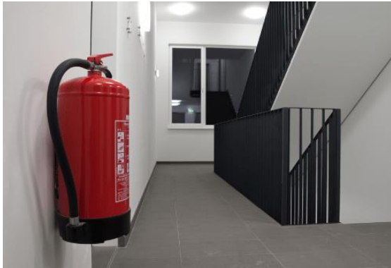
Figure 5: Installation of appropriate fire-extinguishers
