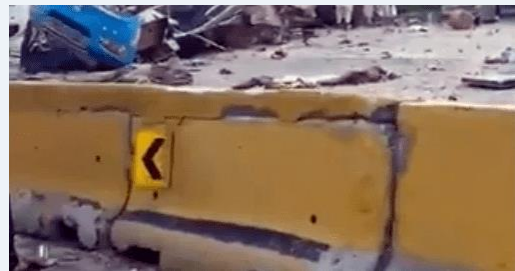
Figure 5: Median barrier of motorway
