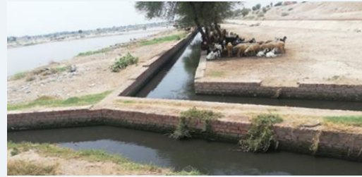
Figure 10: Northern waste water treatment plant
