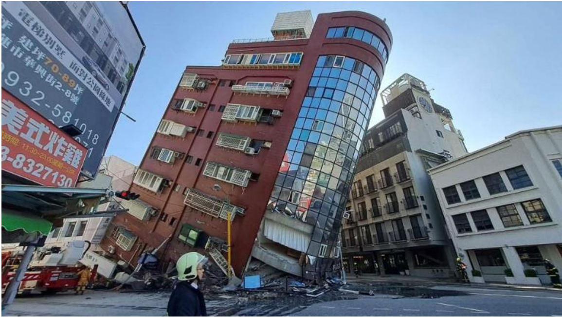
Figure 1: A building in Hualien, Taiwan leans dangerously after a magnitude 7.4 earthquake on 3 April 2024. Credit: VCG via Getty
