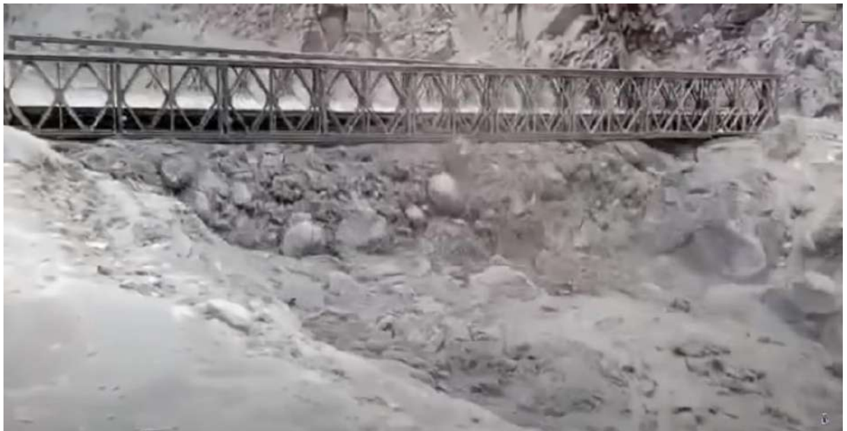
Figure 11: Frame-8 Bridge very far away from the original position and about to lose its support on earth
