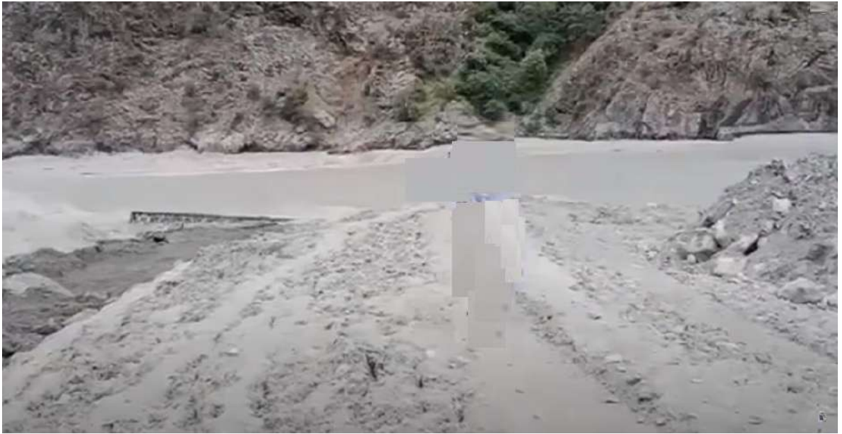
Figure 13: Frame-10, Bridge afloat in water, with its top partially visible
