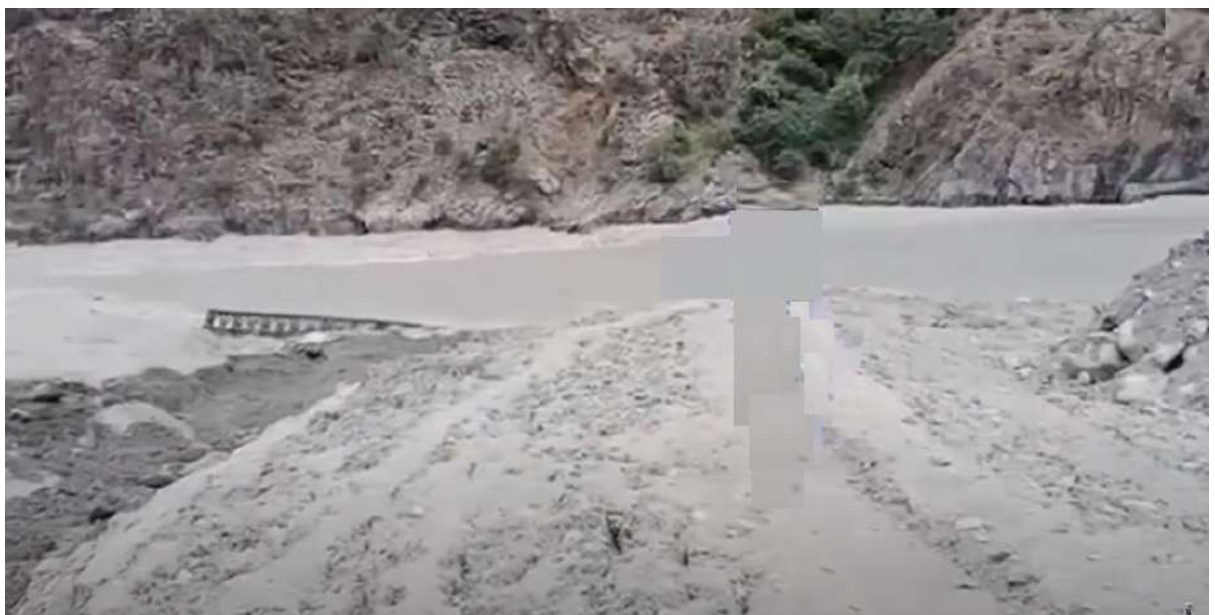
Figure 12: Feame-9, Bridge afloat in water
