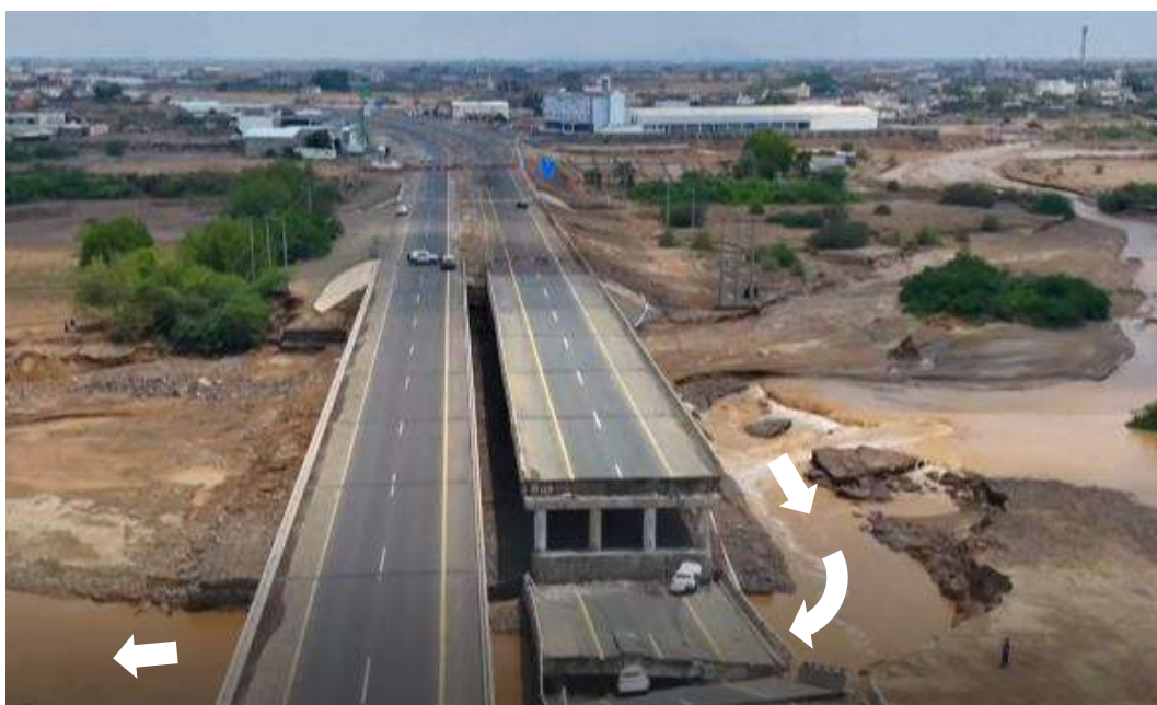
FIGURE 4: A PERSPECTIVE VIEW OF THE COLLAPSED BRIDGE
